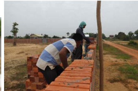
Finishing building 130cm high of wall
